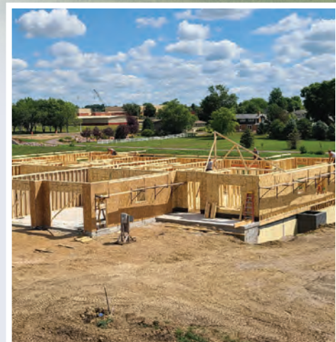
Check out the new UITHOVEN ADDITION near Luverne Public Schools and the Luverne Loop!
