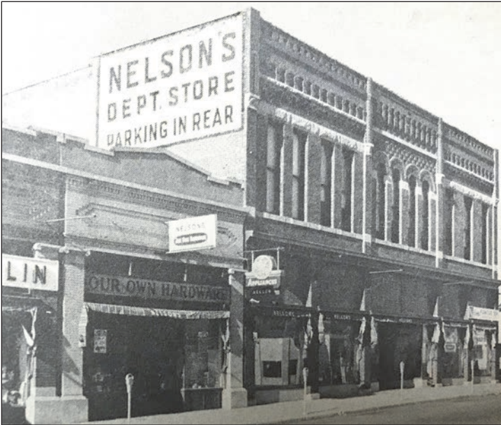
Nelson’s Department Store prior to the 1973 remodel project.
