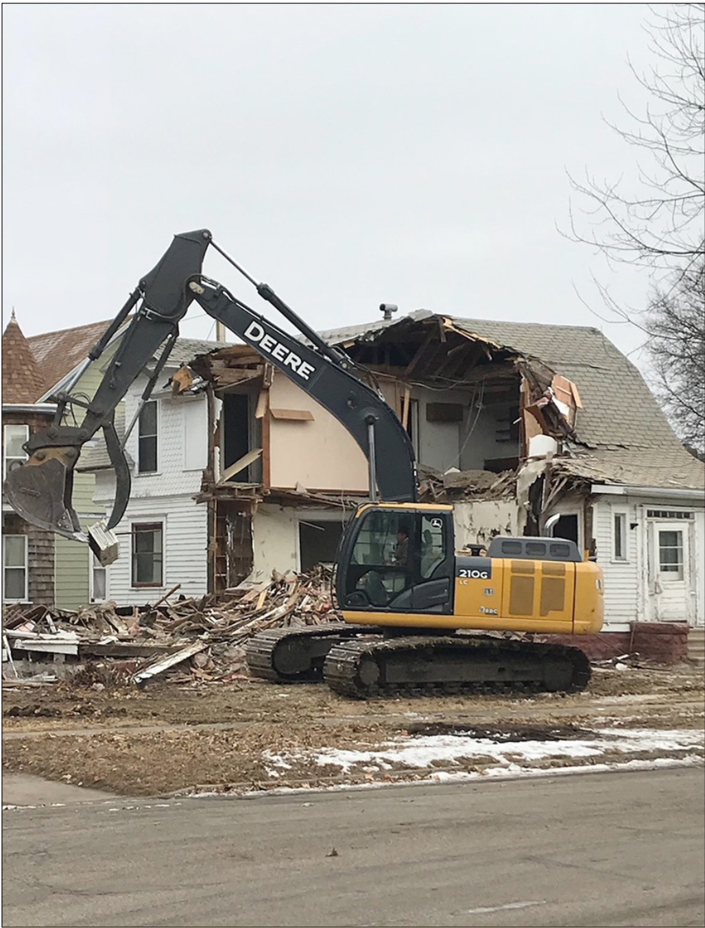
Chantel Connell photo/1214 house demo lincoln and freeman
