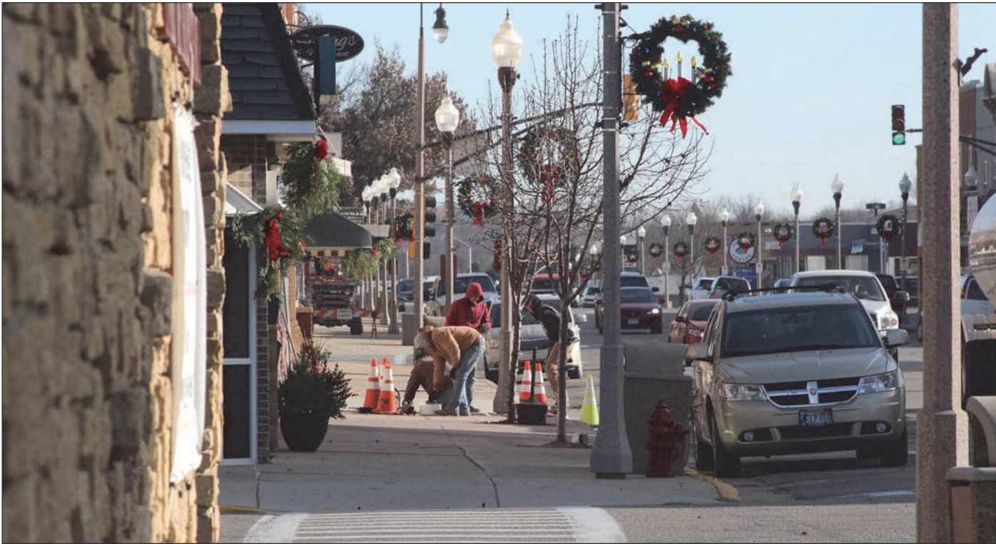
Lori Sorenson photo/1207 wires downtown
