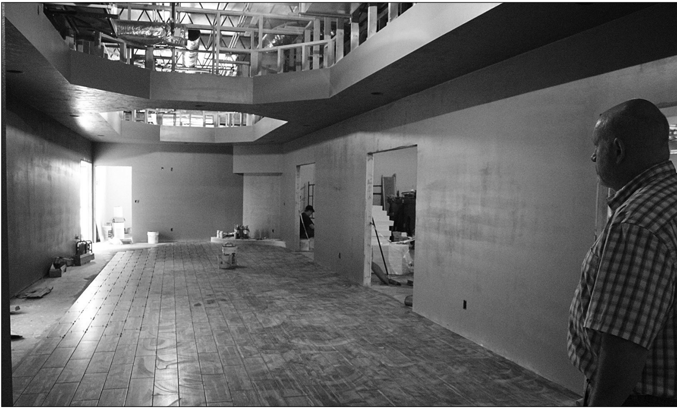
Lori Sorenson photos/0616 grand prairie events center lobby
