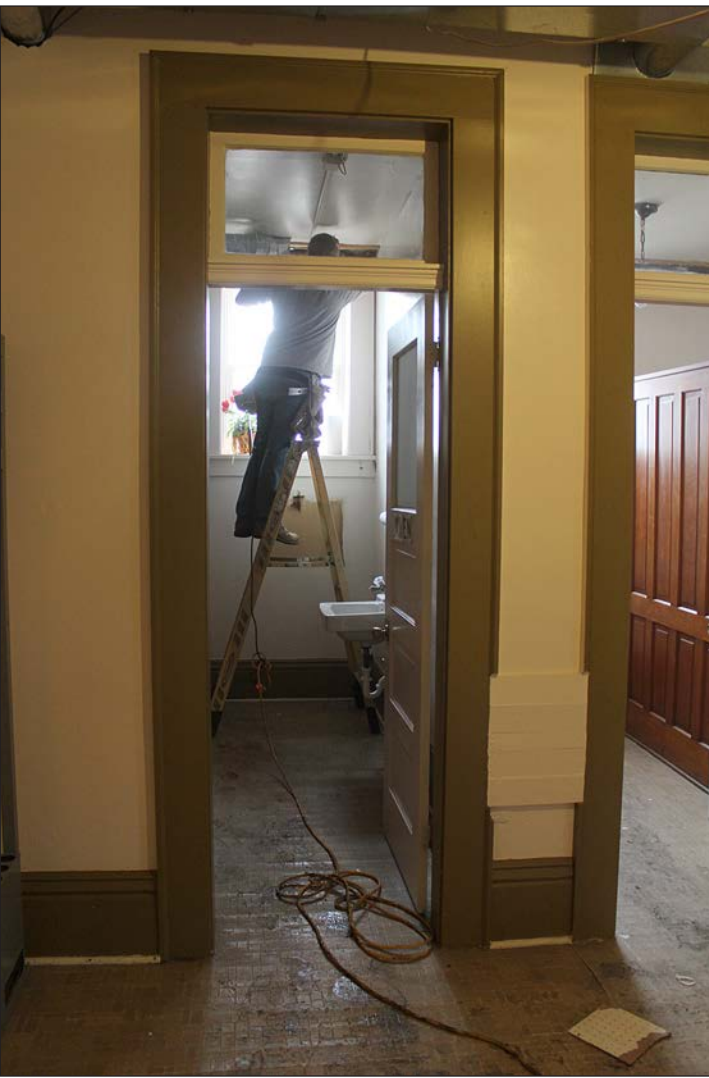
Lori Sorenson photo/0303 carnegie construction
