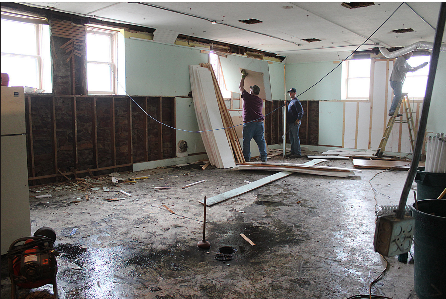
Lori Sorenson photo/0303 carnegie construction
