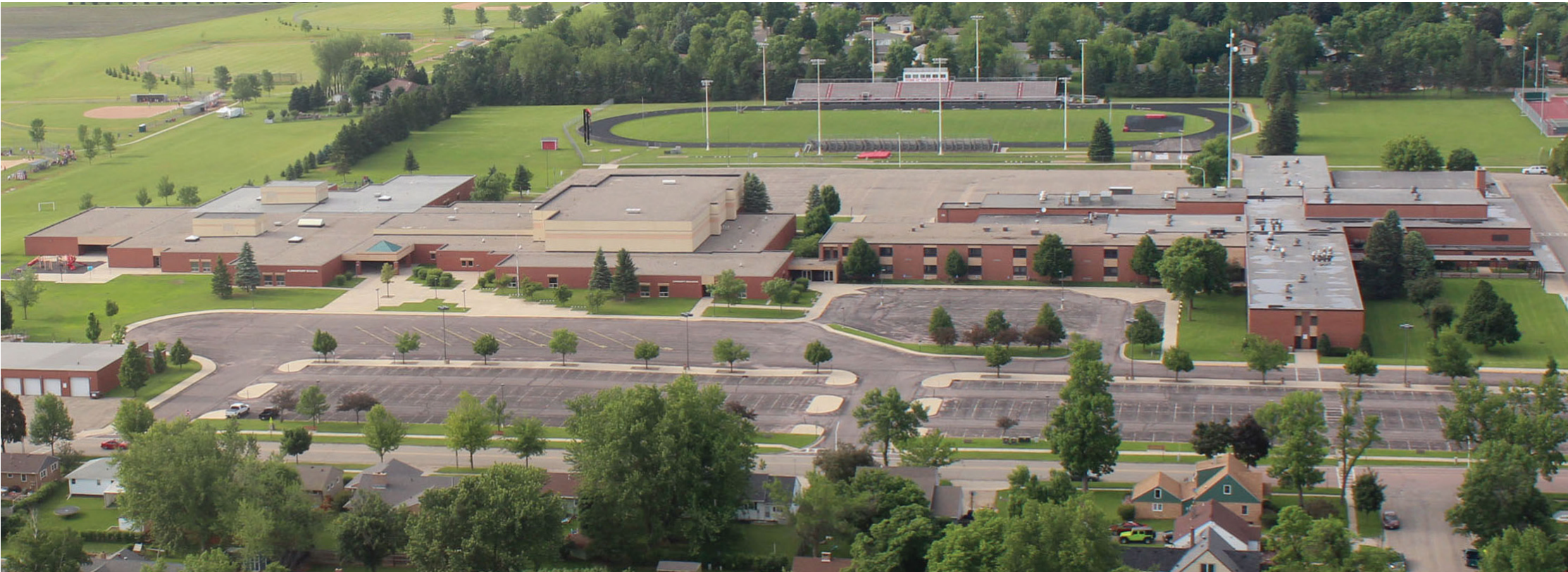
This 3-year-old aerial photo offers perspective on the current south-side view of the Luverne School District parking areas and building footprints to compare to construction plan drawings.
