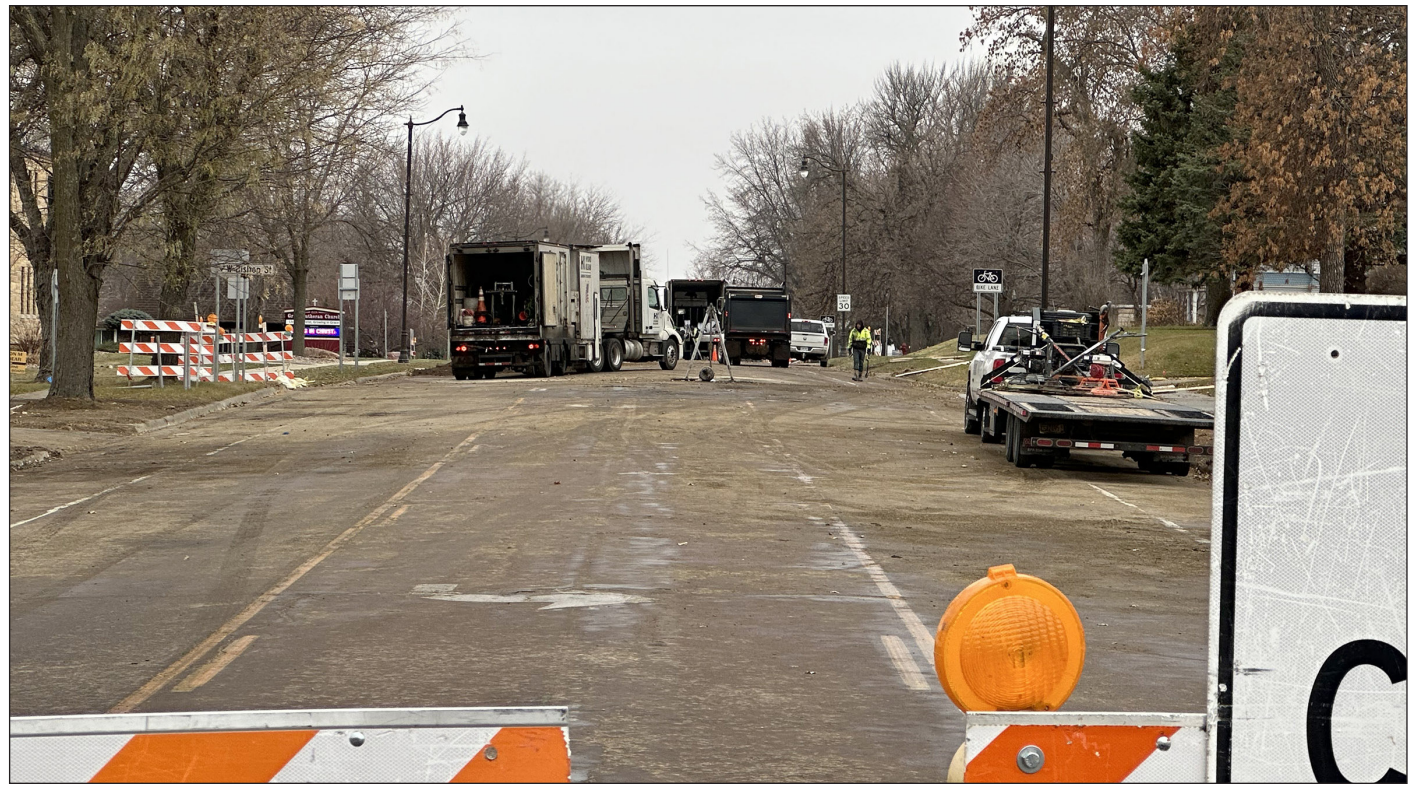
Lori Sorenson photos/1110 highway 75 construction
