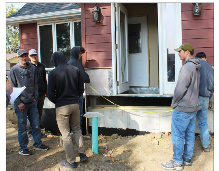
Darrel VanAartson's construction trades class measures for a new two-stall garage and calculates the amount of fill necessary to prevent water flowing to the newly moved house on East Dodge Street.
