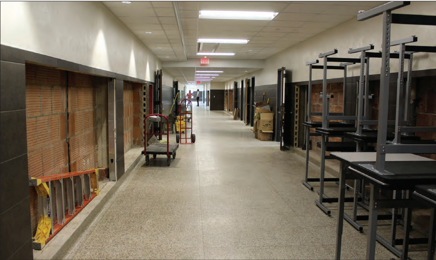
Mavis Fodness photo/0924 School Build South Wing Second Floor
