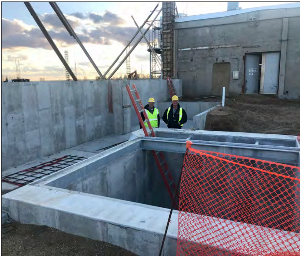
Above, a tour group takes stock of construction activity in the basement activity where rendering and other waste is handled. At left is the start of the CO2 chamber, which is 30 feet deep.
