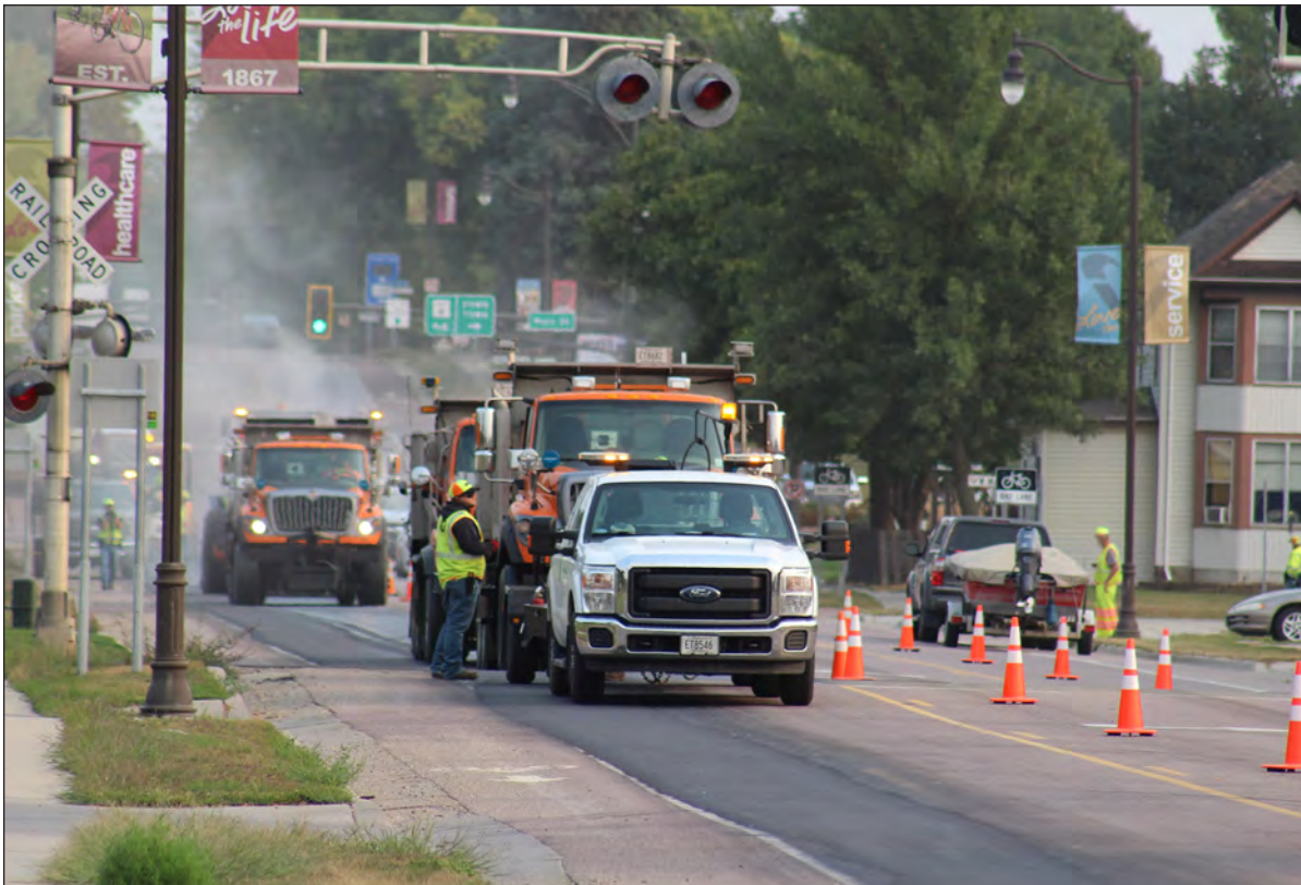
Mavis Fodness photo/0924 Hey 75 Repairs
