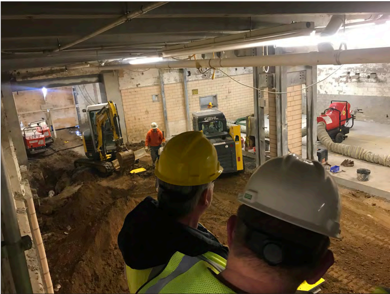
Above, a tour group takes stock of construction activity in the basement activity where rendering and other waste is handled. At left is the start of the CO2 chamber, which is 30 feet deep.
