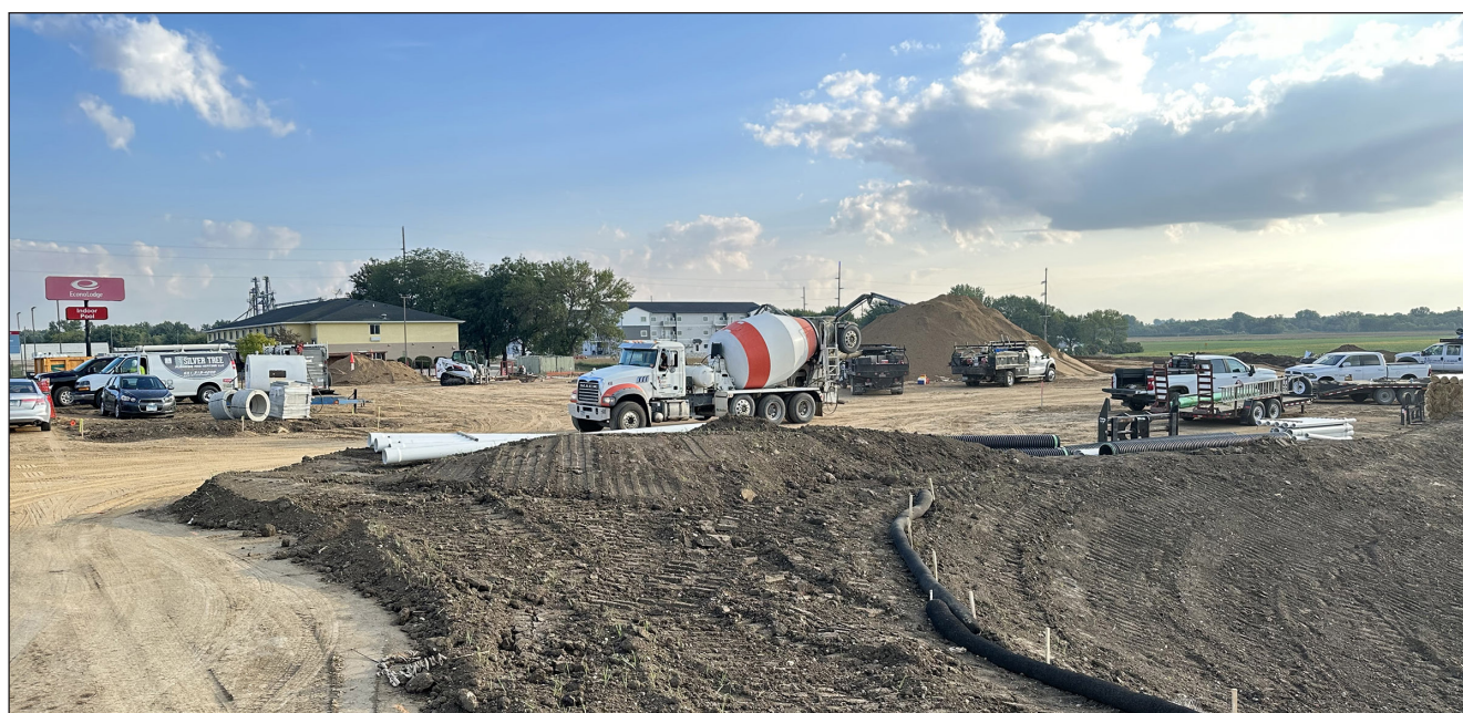
Lori Sorenson photo/0921 kwik trip construction
