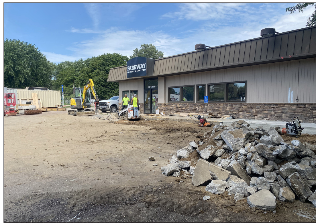
Lori Sorenson photo/0825 fareway meat construction
