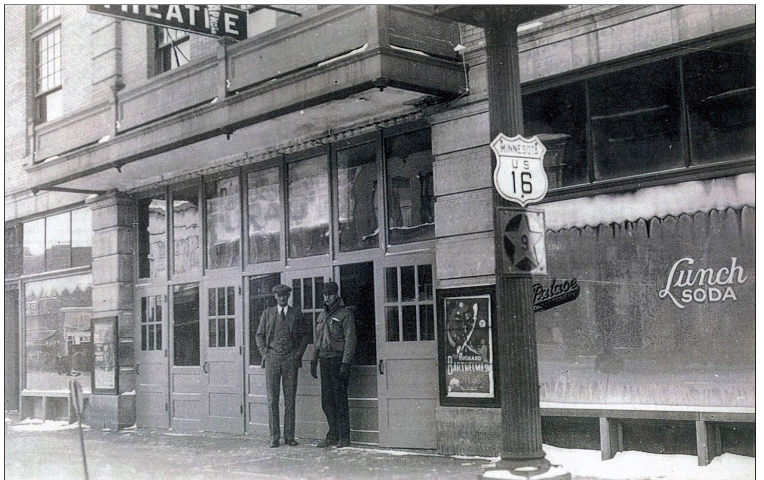
A 1920s-era photograph shows the protective temporary doors on the front of the Palace Theatre in the wintertime.
