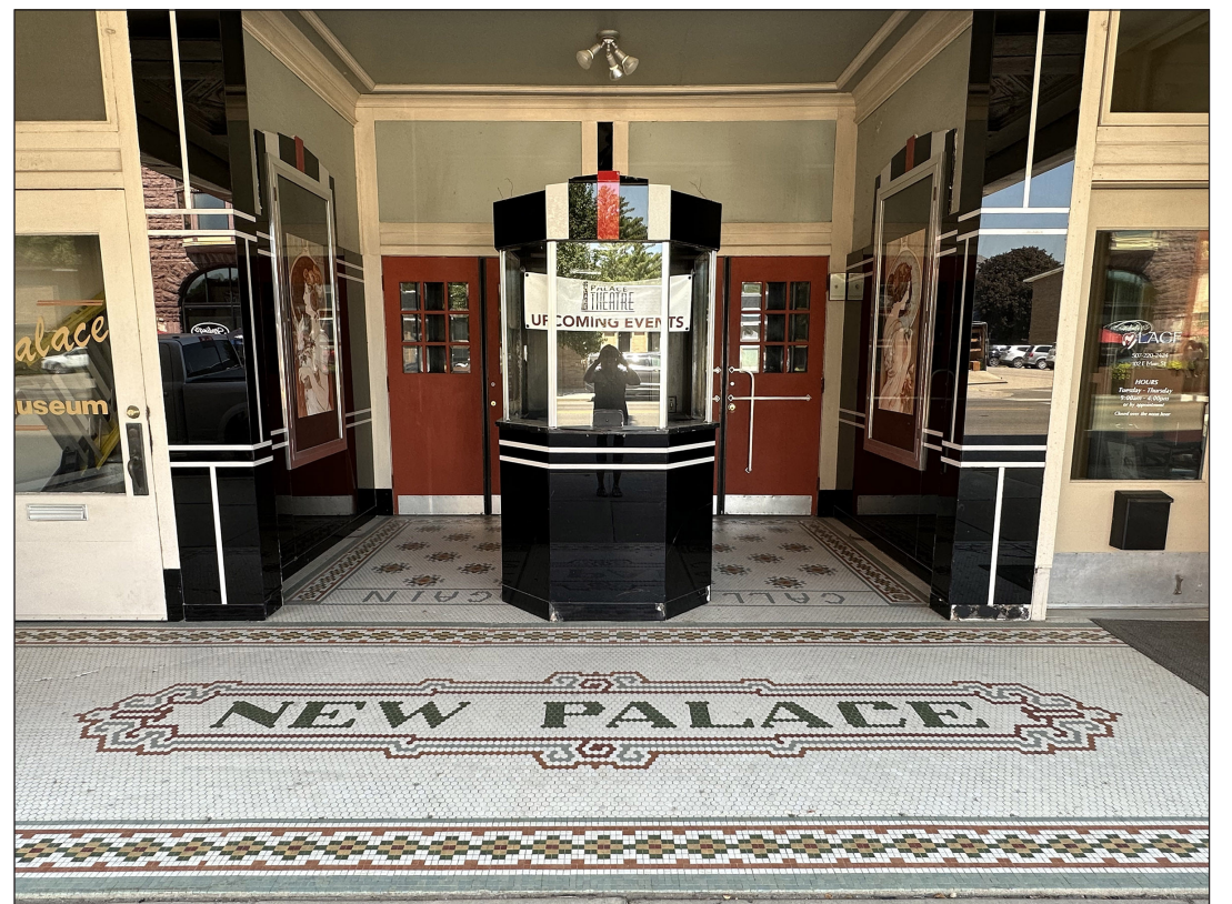
A current-day image of the Palace Theatre shows the historic tile flooring and recessed entry way that is open year-round. Below left is an architect’s rendering of what the remodeled Palace entry will look like. Below right is an image of the original doors that once served as the theater’s temporary entry erected in the winter time.
