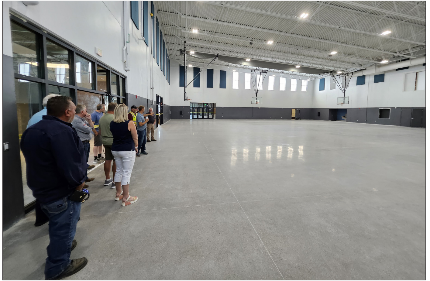
Above, the assembly hall (or drill hall) is the main space for the readiness center and will be available for community use. Below right, classrooms and work spaces include full technology access and ample natural light.
