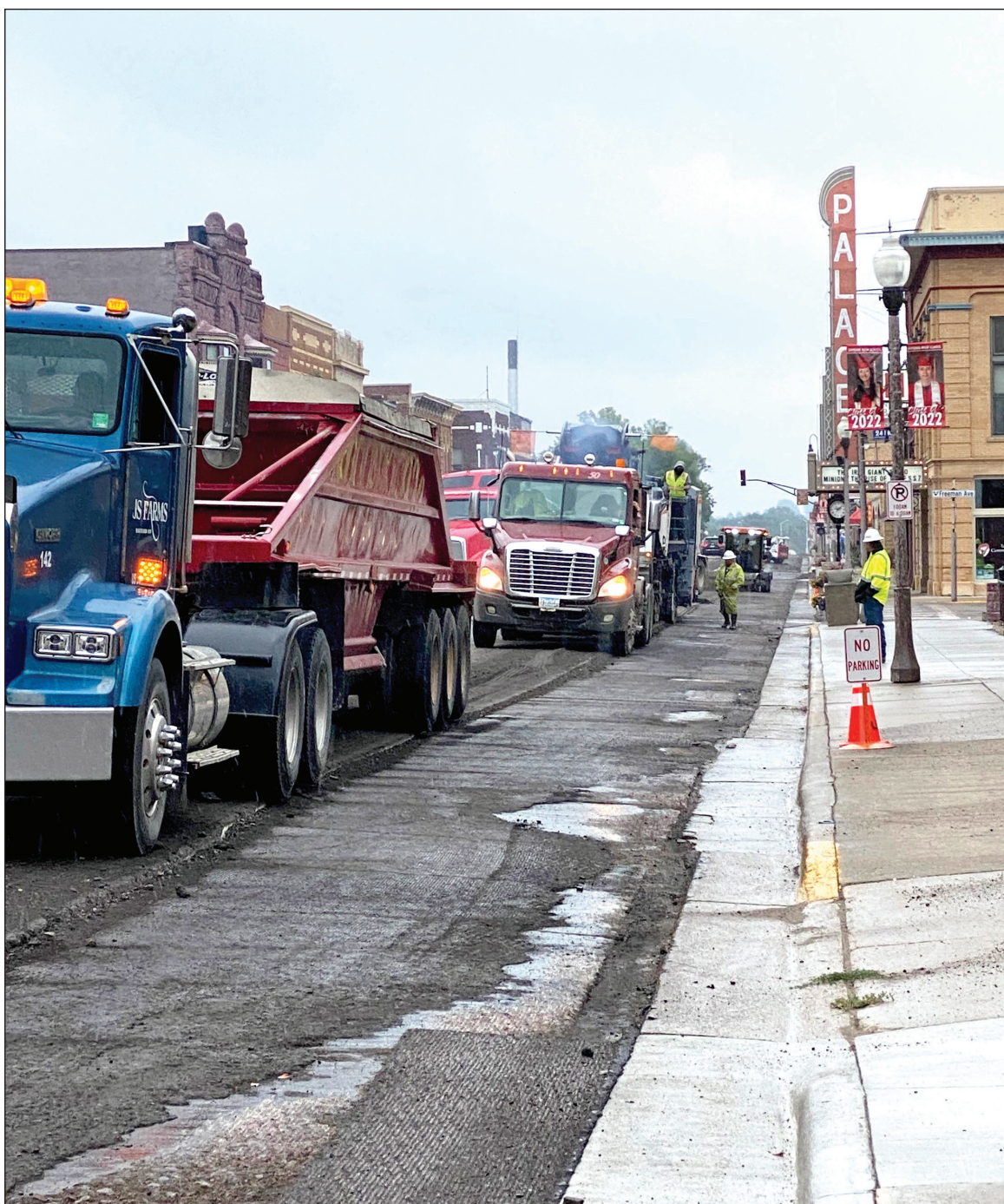
Lori Sorenson photo/0818 road construction
