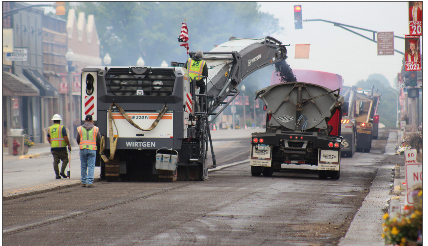
Mavis Fodness photo/0818 road construction
