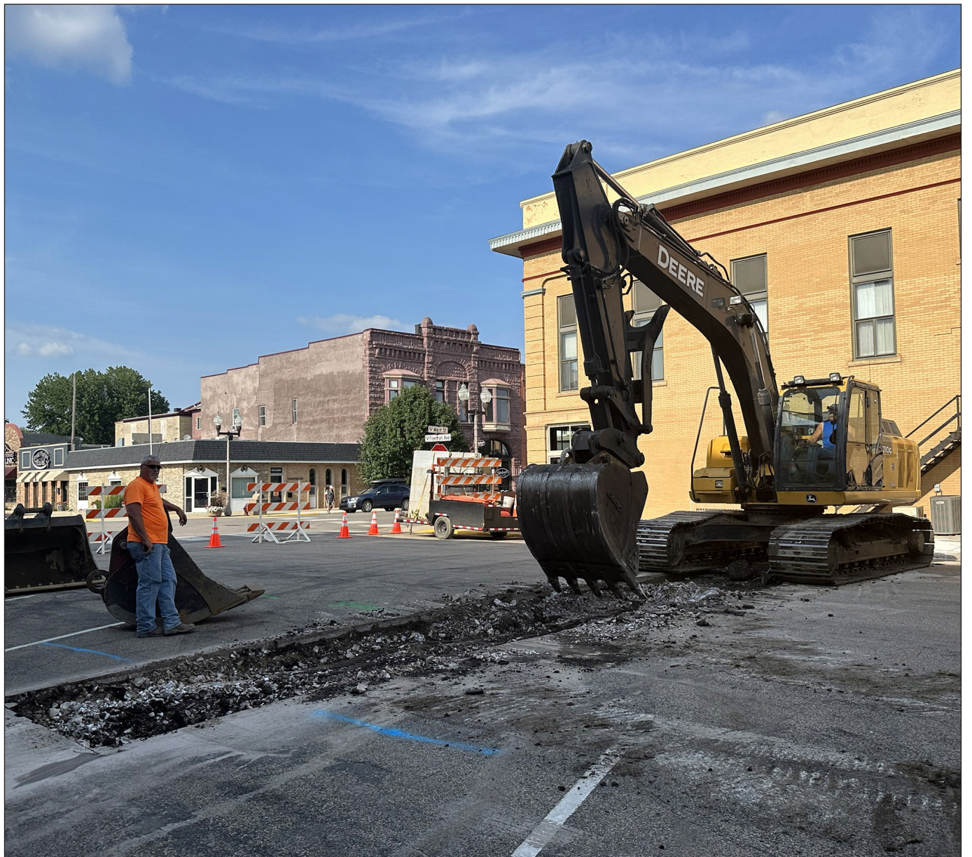
Lori Sorenson photo/0810 freeman ave work near palace theatre
