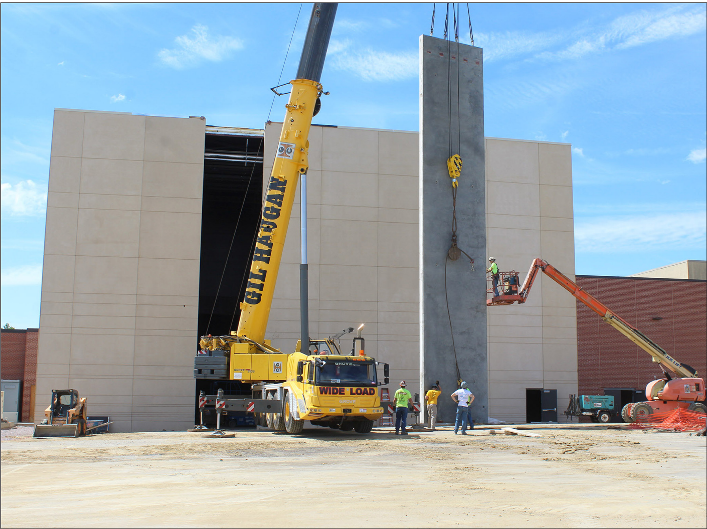
Mavis Fodness photo/0701 School Build Last Panel
