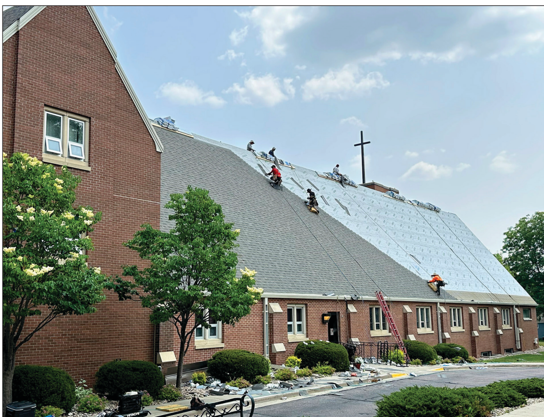
Lori Sorenson photo/0622 presbyterian church roof work
