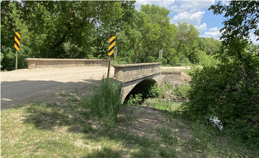
The Spring Brook Bridge is a single-span, reinforced concrete, filled-spandrel, barrel-vaulted, arch bridge, with slightly flared wingwall abutments. It was constructed in 1911 by Perley N. Gillham, who designed and constructed reinforced-concrete arch bridges. (Lori Sorenson photo)
