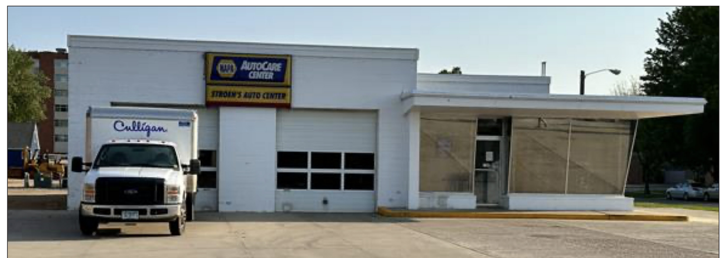
Culligan is moving into the former Stroeh's Auto building on East Main Street, and the Luverne Economic Development Authority is helping with some exterior improvements through the city's facade improvement program.
