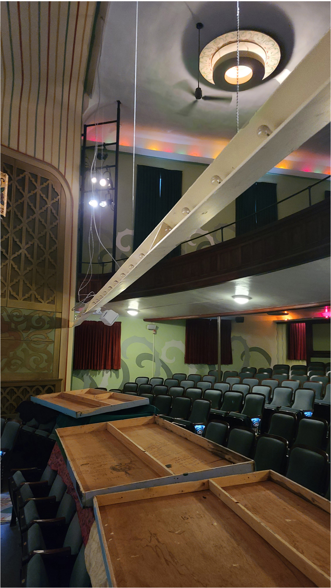
A light bar from the ceiling is lowered to replace bulbs, one of several maintenance items Palace Theatre staff tackled during downtime of the pandemic shutdown. According to Palace director Shawn Kinsinger, the bulb replacement was a complicated process that involved climbing through a hole in the ceiling of the apartment upstairs to get to the pulleys that lower the light bar.
