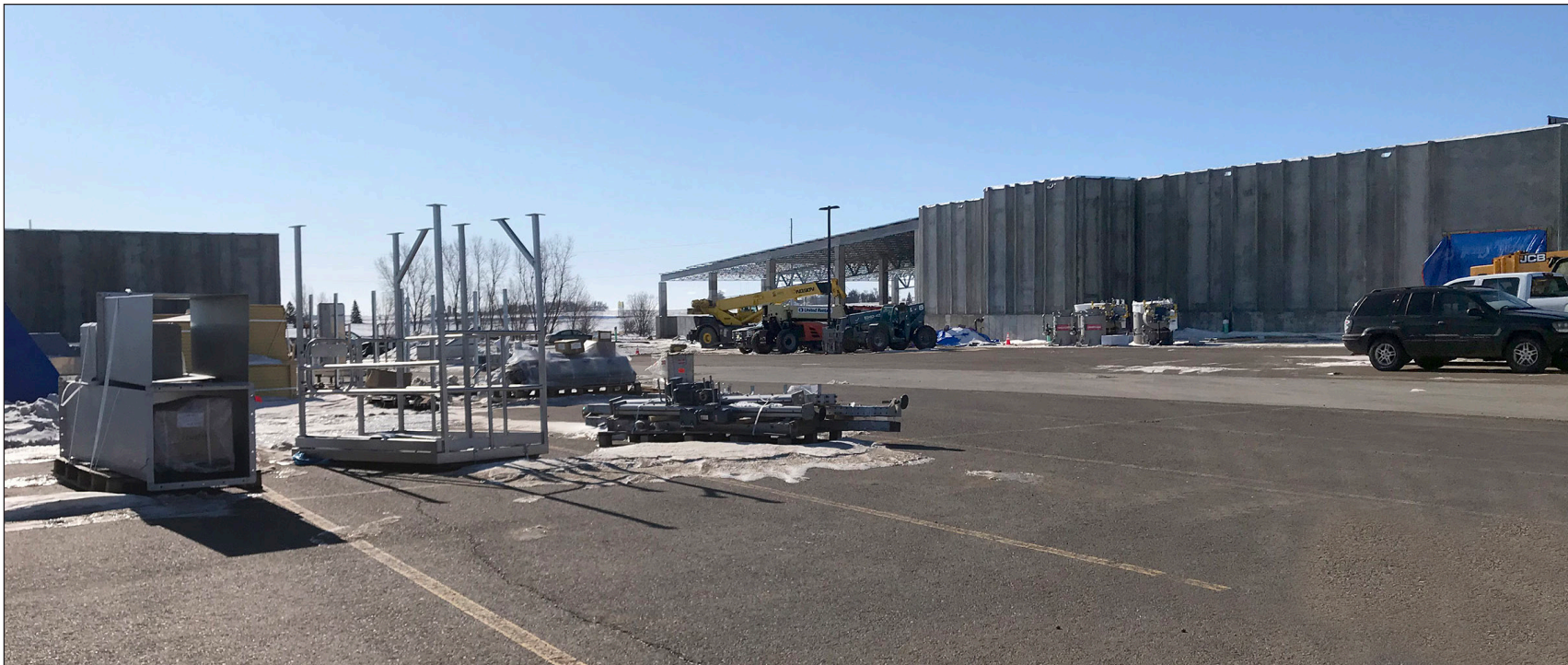
Premium Minnesota Pork is nearing completion on its $30 million expansion and retrofit of the former Gold'N Plump facility on the west edge of town.
