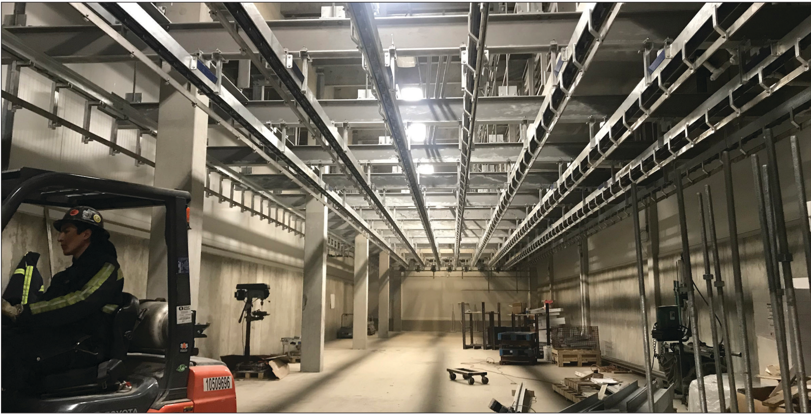
The coolers represent about 17,000 square feet of the 128,000-square-foot plant, and they involve the most automated aspect of production. The coolers are divided into two bays, each with 100-foot-long rails designed to carry a total of 2,500 hogs. (Lori Sorenson photos)
