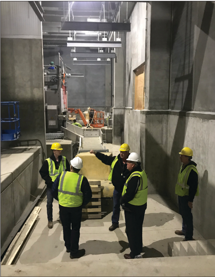
As Premium Minnesota Pork nears completion on its $30 million construction, President Dan Paquin is leading more frequent tours.
