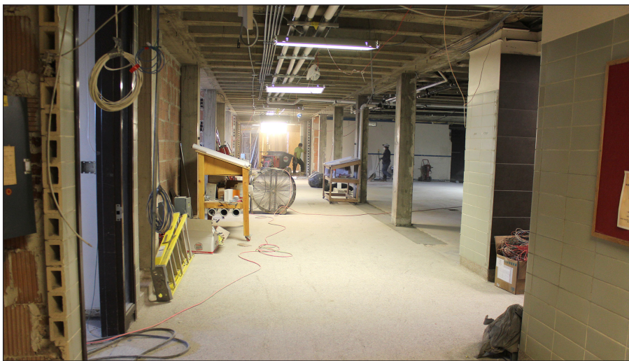
Workers began demolishing the first floor of the Luverne Middle-High School west wing (including the superintendent’s office) recently and, as of Friday, were almost complete. This is a look down the hallway, facing west.
