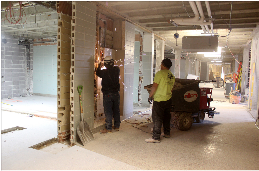
Gil Haugen workers remove tile from the front of the former bathrooms on the first floor of the west wing. This picture is taken facing east.
