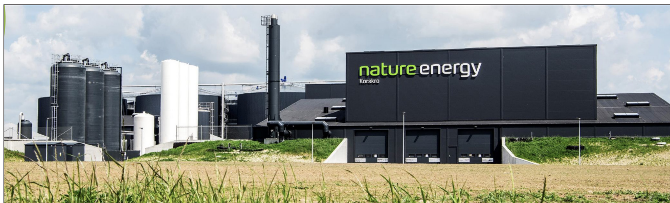
The company extracts methane from cattle manure and other organic wastes to produce biogas, which is sold as a green alternative to natural gas. The manure, minus the gases, is returned to the livestock producer as fertilizer.
