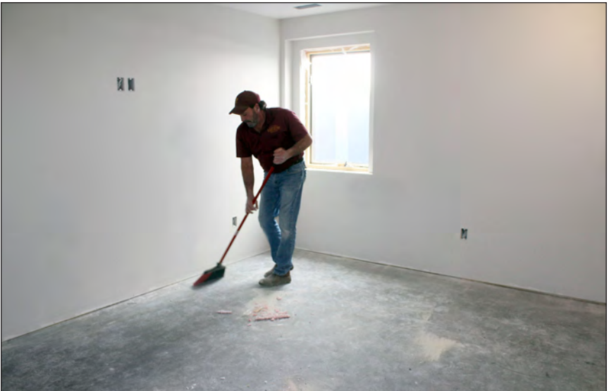
Greg Uithoven cleans the floor in one of the basement bedrooms. The new home will have four bedrooms and three bathrooms.
