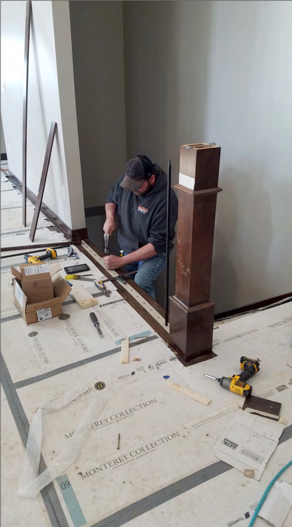
Adam Uithoven installs the stair spindles to allow more natural light to reach into the basement stairs and family room. (Submitted photo)
