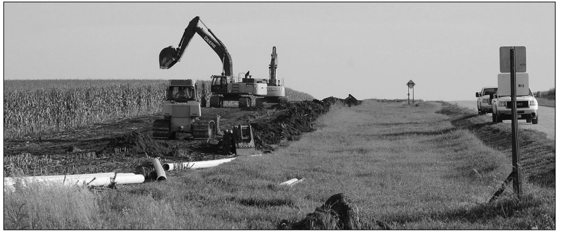
Lori Sorenson photo/0910 rural water construction
