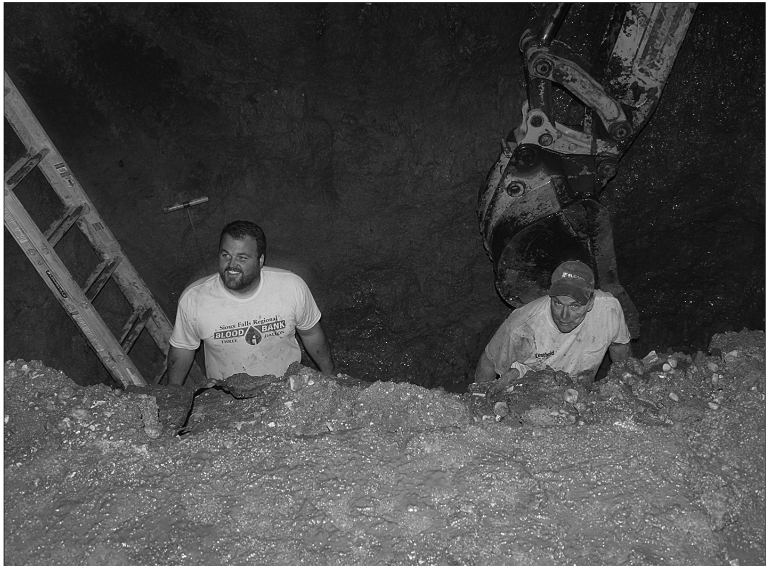
Glenda McGaffee photo/0421 water pipe repair
