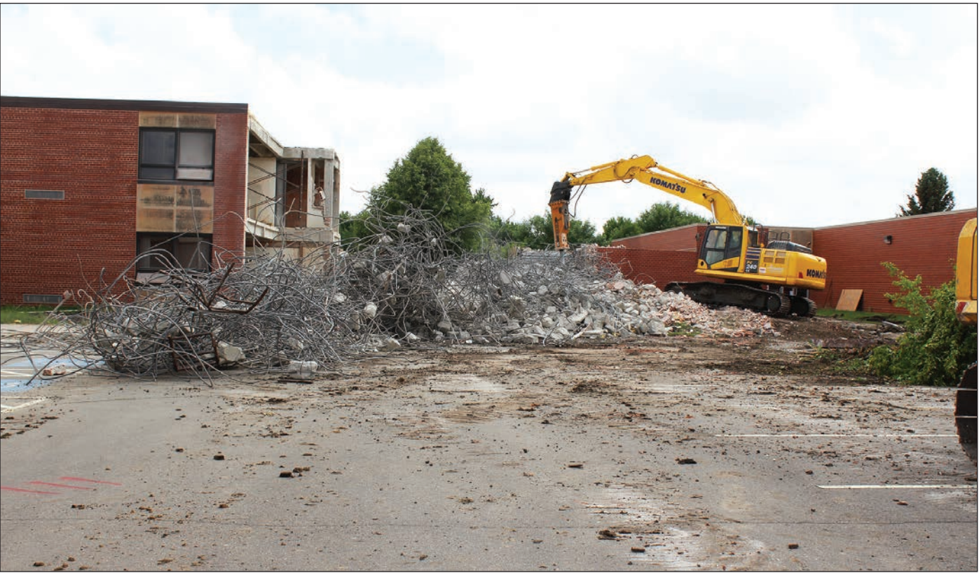
Mavis Fodness photo/0627 School Demo June 19 Demolition June 19 exposes the vast amount of steel reinforcement used in the cement framing of the middle-high school.
