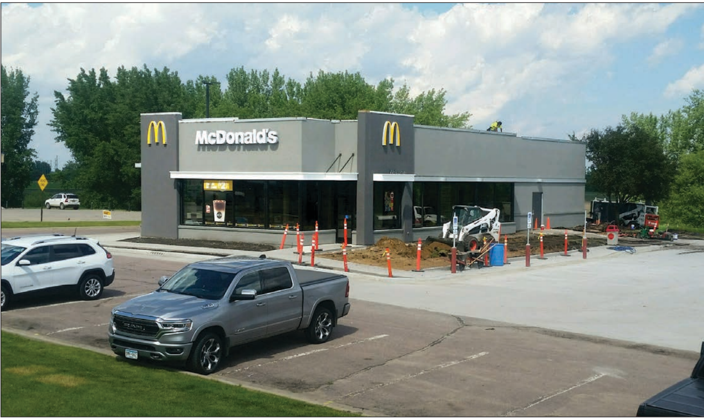
Jason Berghorst photos/0627 McDonald's improvements
