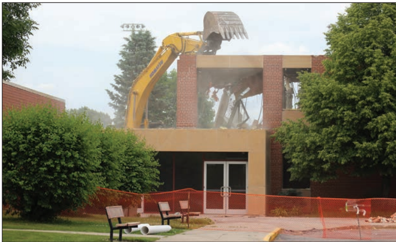
The excavator reaches over the top of the breezeway between the elementary and middle-high school facilities. This photo was taken Thursday, June 20, from the south parking lot facing north.
