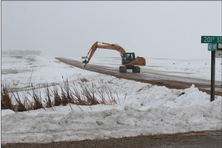
Mavis Fodness photo/0321 Flooding March 14 Chad Ver Steeg uses an excavator to remove snow from ditches on the east side of Hardwick to prevent water from flowing over the roadways.
