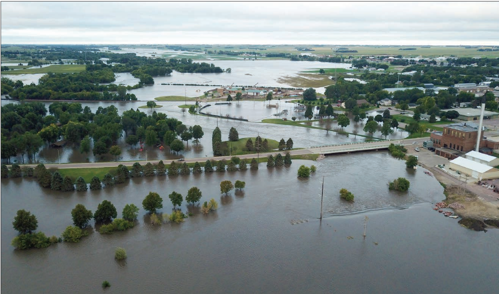
Luverne drone operator Ryan Gee shared this image of East Main Street and Luverne's City Park under a flooded Rock River Thursday.
