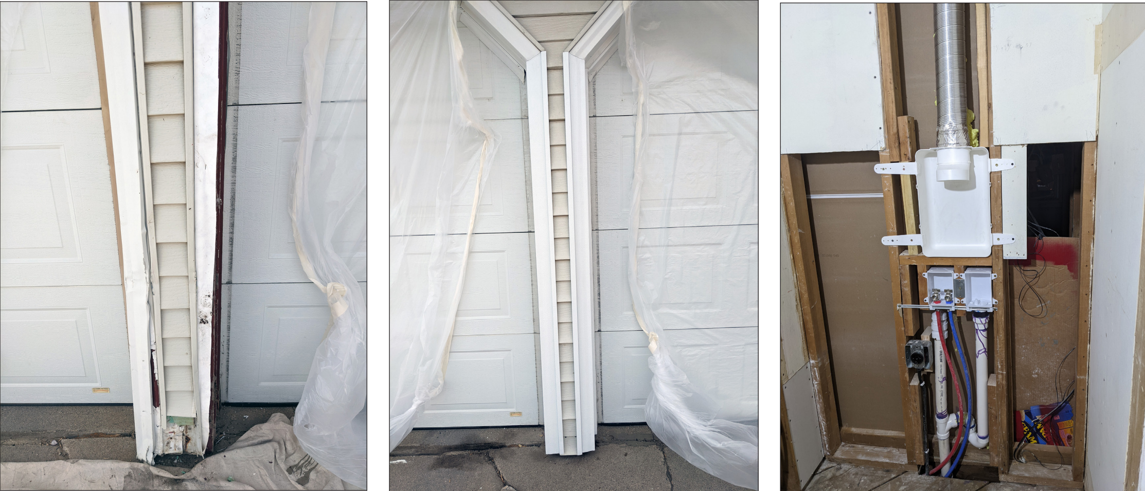
Accidents happen, and M & Em Handyman is able to make repairs (above left and center) and improvements. (Above, right) Matthew Sterrett began improving his own rural Hardwick home to include an upgraded laundry area and remodeled bathroom (pictured below, right). The two improvements are examples of projects he and his fiancée Emily Bassett are willing to complete for other homeowners as part of their new business, M & Em Handyman.
