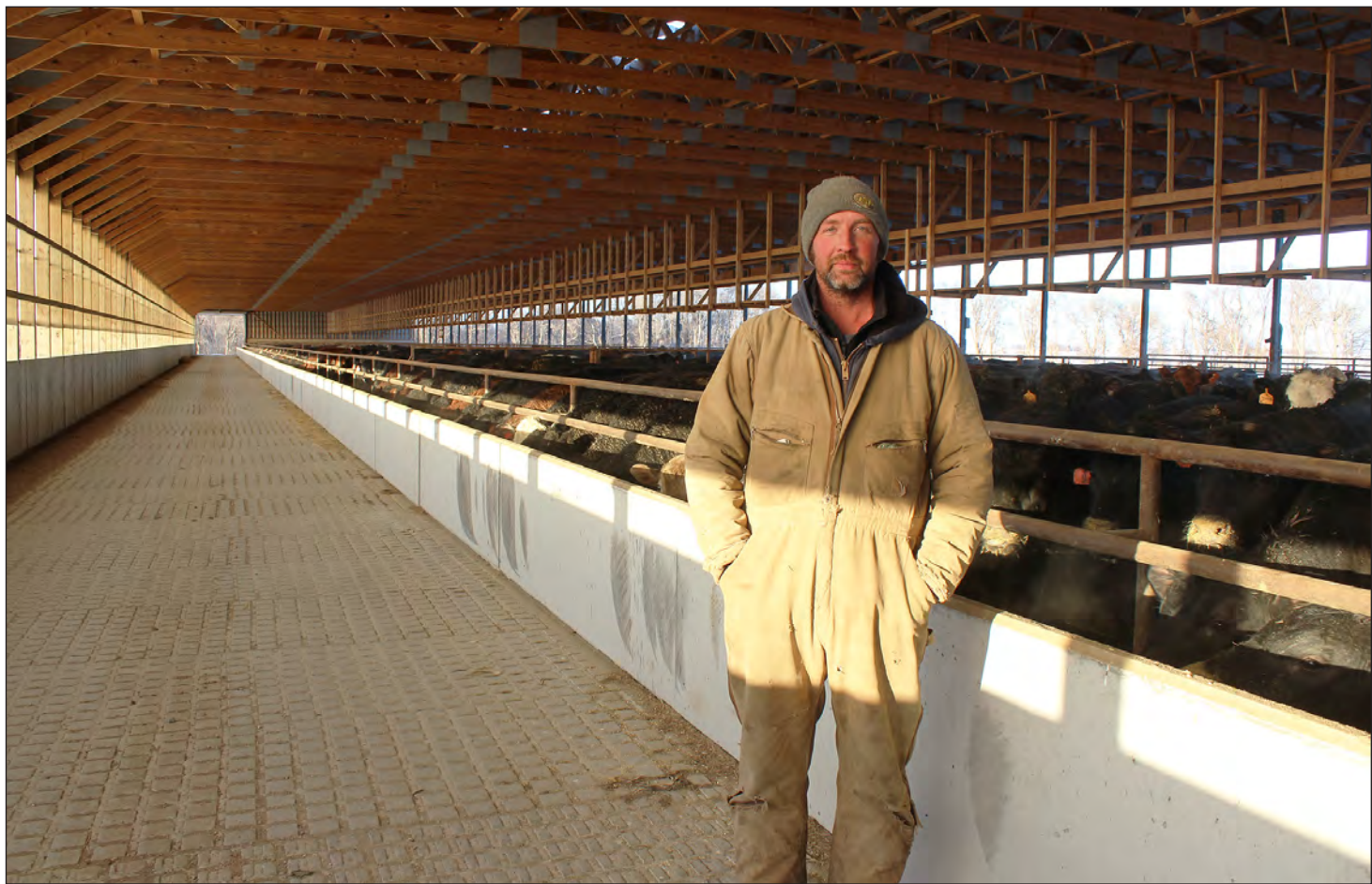
Mavis Fodness photo/0225 Ag Tab 2021 Sandbulte Mike Sandbulte stands inside the new full-roof cattle barn, which allows livestock protection from the weather extremes. The barn, built in 2020, is not fully enclosed to promote good ventilation for the stock that have full winter coats that protect them from the extreme cold. Daily chores in the barn consist of making sure the stock is fed twice a day. No bedding is needed, and manure removal is necessary only once a year. Below , Sandbulte loads feed for 1,800 head of cattle east of Hardwick.
