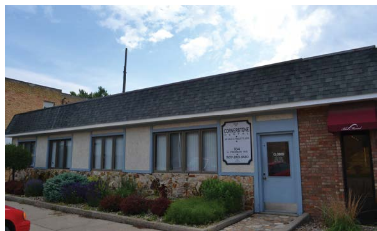
The Rock County Eye Clinic is expanding into the former dental office next door to the north. The graphic below shows what the front will look like when finished.
