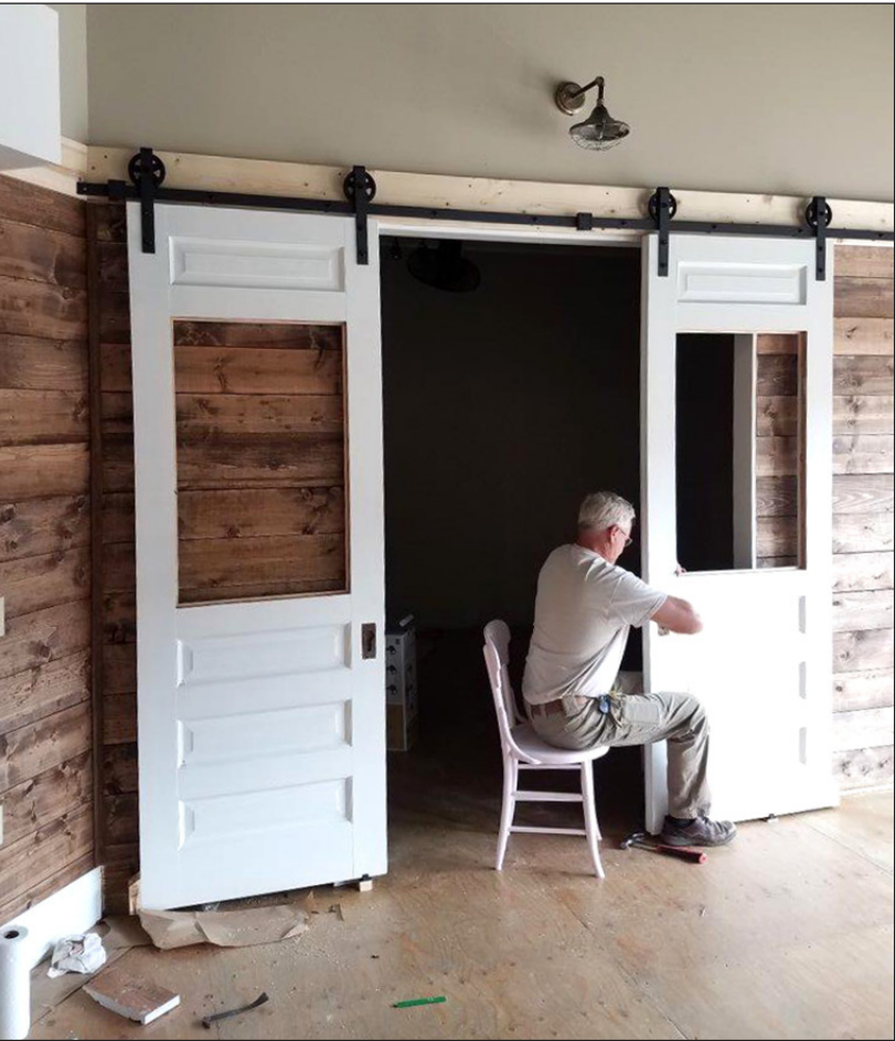
At left, Curt Valnes recycles doors from upper floors of Sterling's (Arcade building) for a "barn door" entrance to ComputerTutors in the Mall on Main. (Above) the original Nelson Bros. pillars were uncovered, painted and incorporated into the interior decor.
