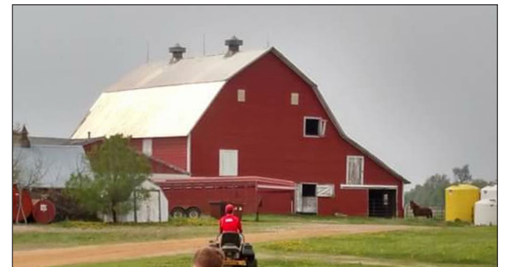
This photo of the Van Meeteren barn was taken this spring.
