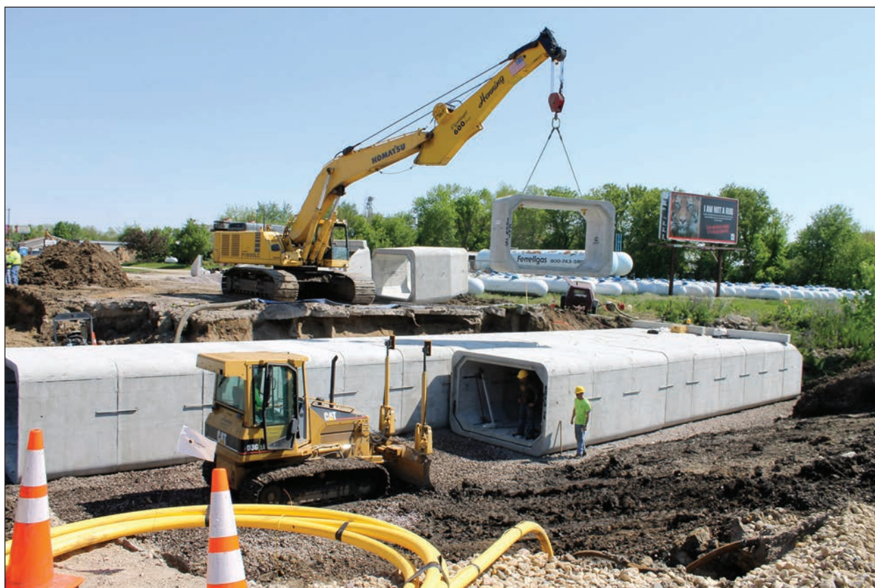
Mavis Fodness photo/0528 Hwy 75 culvert
