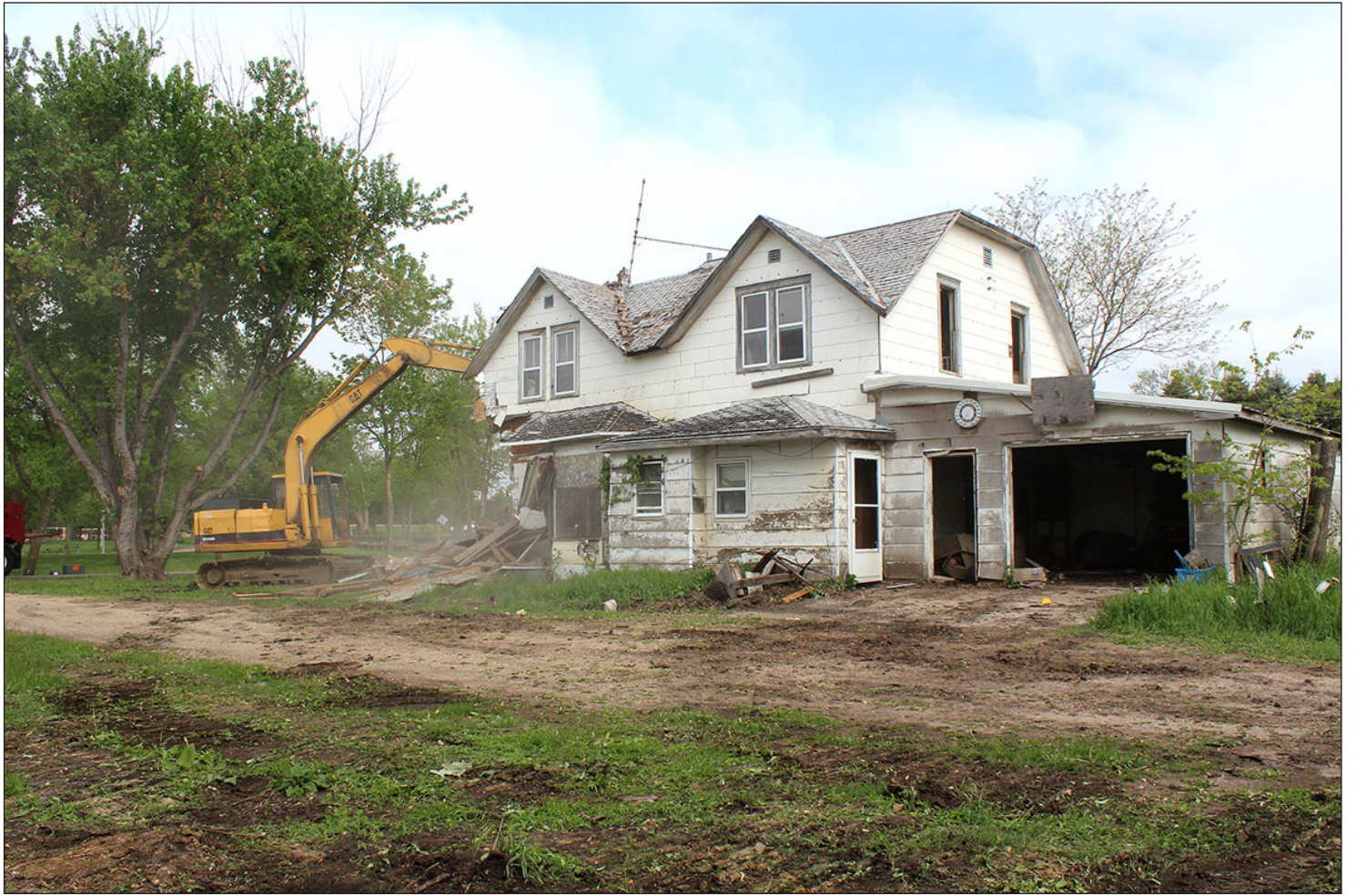
Stephanie Christensen photos/0528 sterrett demolition
