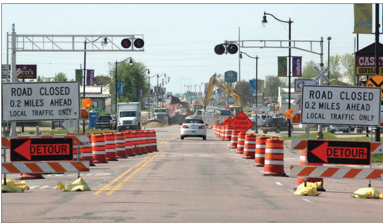
Lori Sorenson photo/0521 highway 75 construction
