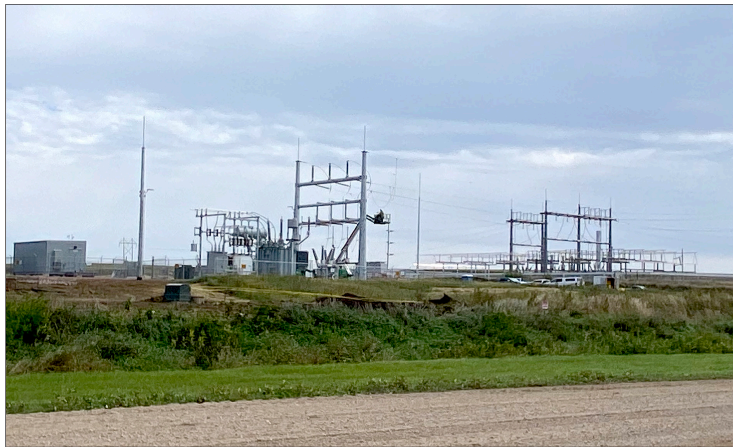
Every single turbine has buried cables — collection lines — that take the power they’re generating and send it back to NextEra’s collector substation, which collects all the power from the turbines and steps it up to a higher voltage and sends it to a “point of interconnection” substation owned by Northern States Power, which then sends it the grid. This 5-acre piece of land is the site of the collector substations and the future operations building where wind technicians will work.
