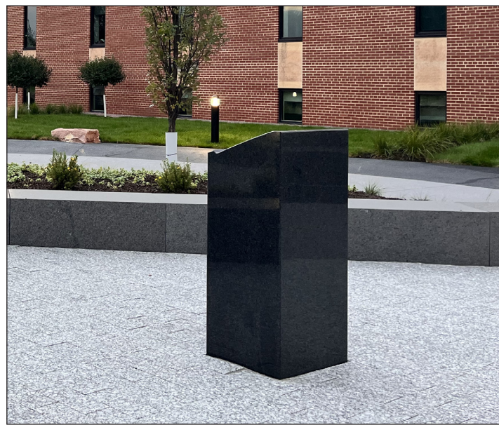
The base of the Alumni Garden includes 154 tons of granite slabs, and Sioux quartzite boulders are primary accent pieces throughout. “It was going to have some dyed concrete, but most of it was going to be regular gray concrete,” said Steve Selseth of Oh’Landscapes. “Now it’s all real granite – regular poured concrete and then a layer – a topping – of real granite mixed into the blend of the topping.”
