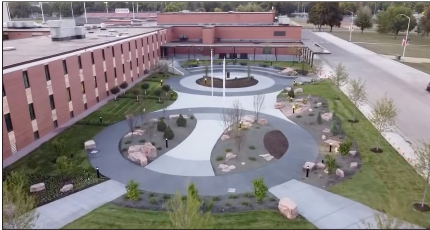
The Luverne Alumni Garden features an amphitheater with stadium seating for 30 to 40 people, complete with a podium and sound system.
