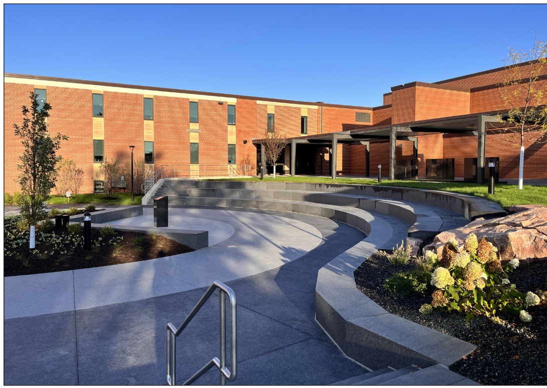
The base of the Alumni Garden includes 154 tons of granite slabs, and Sioux quartzite boulders are primary accent pieces throughout. “It was going to have some dyed concrete, but most of it was going to be regular gray concrete,” said Steve Selseth of Oh’Landscapes. “Now it’s all real granite – regular poured concrete and then a layer – a topping – of real granite mixed into the blend of the topping.”
