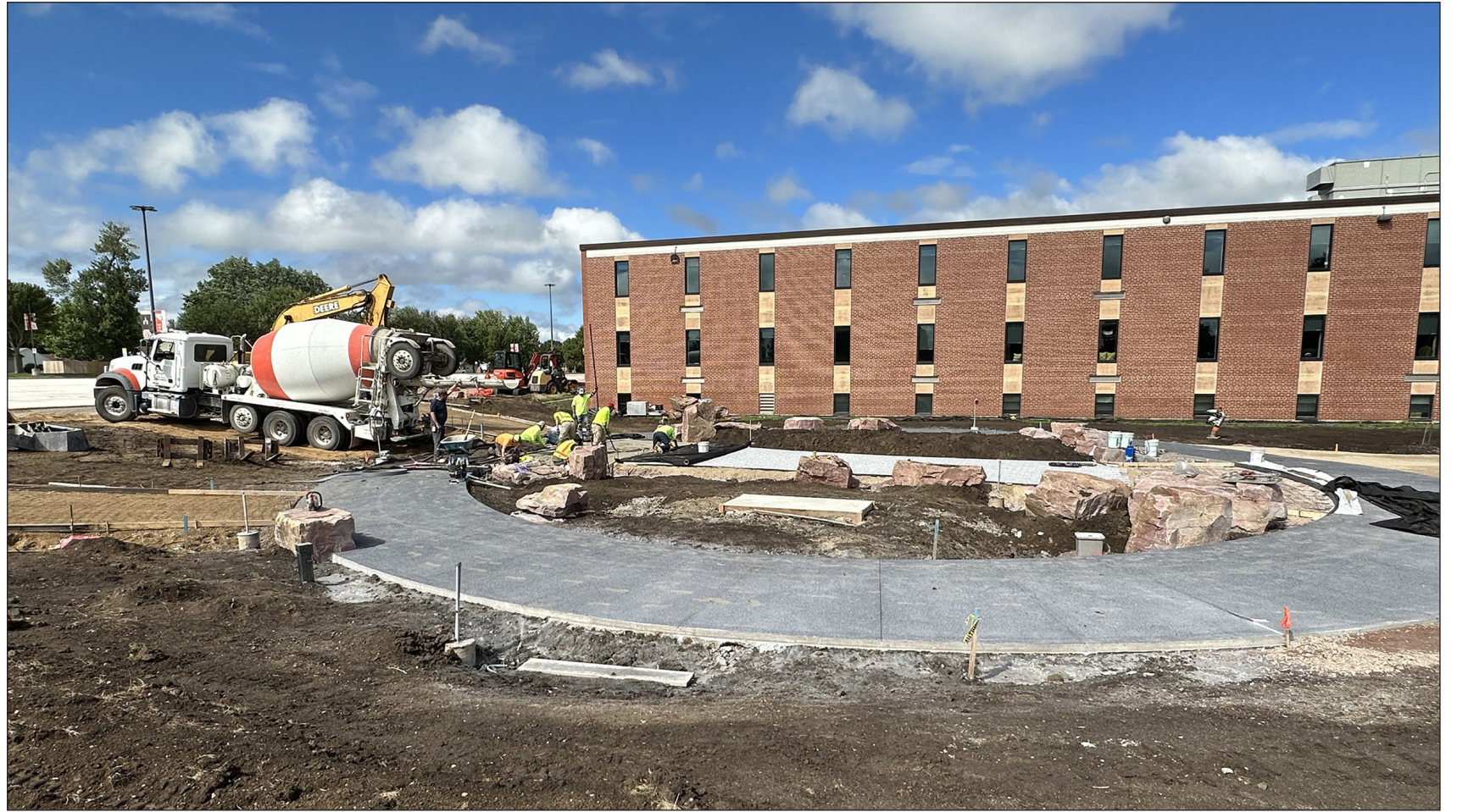
Lori Sorenson photos/0817 Luverne alumni garden construction site
