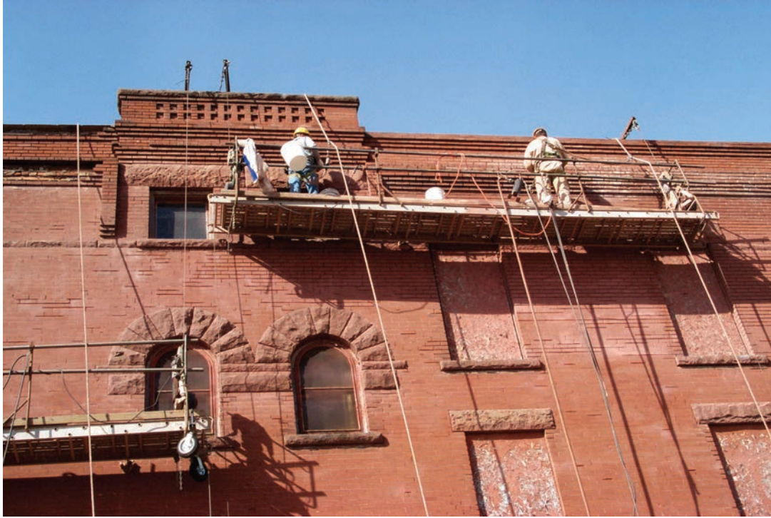
Above and at right, crews work on tuckpointing the Manitou exterior in 2002.
