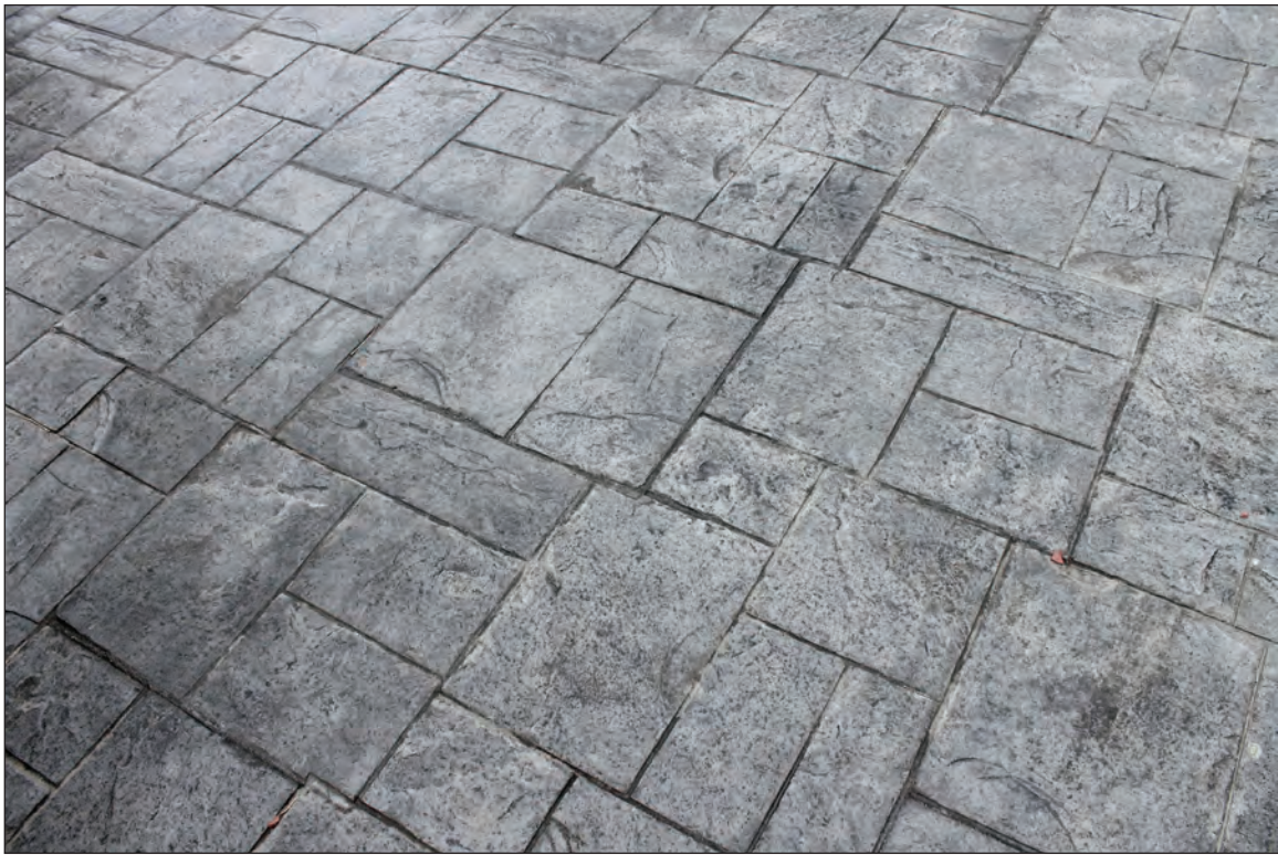
Stamped concrete is able to mock the chisel marks and give the appearance of individual slate bricks. A coloring agent was also added to the concrete, giving it the dark gray look of slate.
